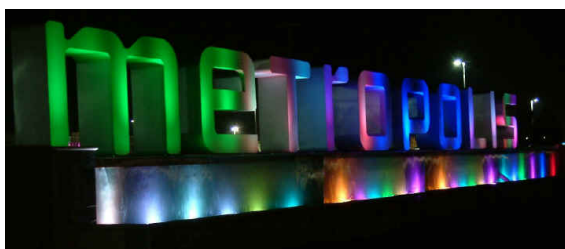
Figure 6. Metropolis Mall Entry Feature 100 foot 2800 GPM waterfall with color changing LED fixtures on eight foot letters. (Plainfield, IN, USA) [11].
